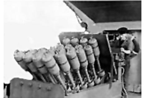
The Hedgehog was an anti-submarine weapon developed by the British Royal Navy during WWII. It was used on destroyers to supplement the depth charge when attacking submarines. It was launched by firing a number of spigot mortar bombs from spiked fittings. Rather than working on a time or depth fuse like depth charges, the bombs detonated on impact and achieved a higher sinking score against submarines than depth charges.
